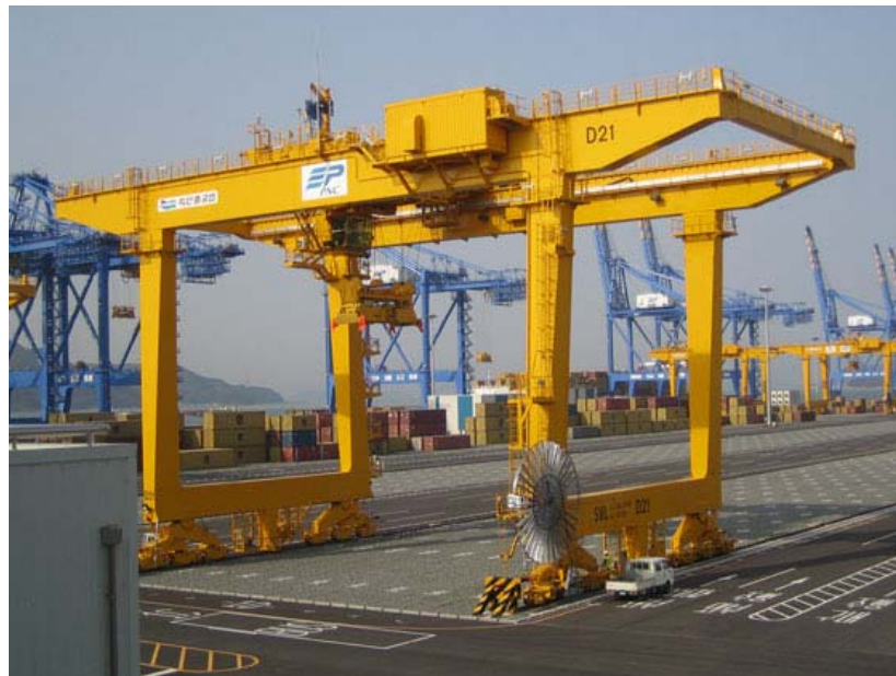
Photo 2: RMG (side-loaded) with Medium-voltage cable reel
